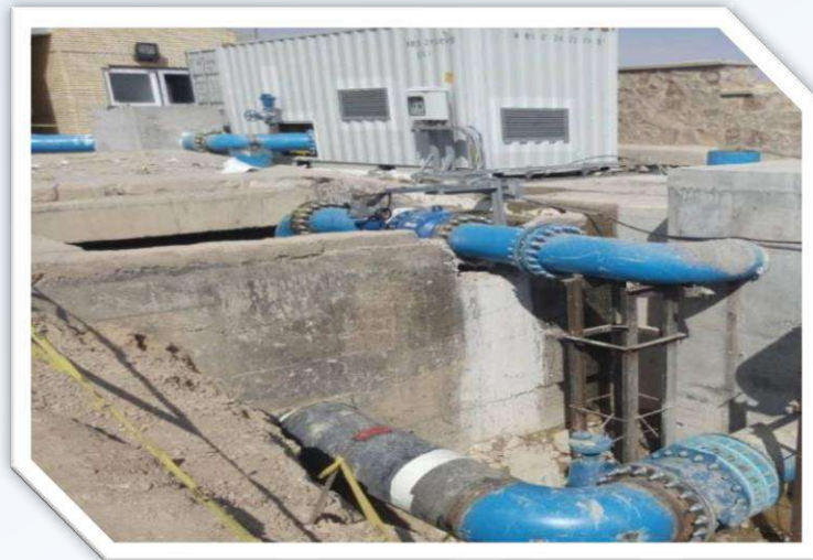
3 MW capacity Small Hydropower (Semnan Province, Iran)
