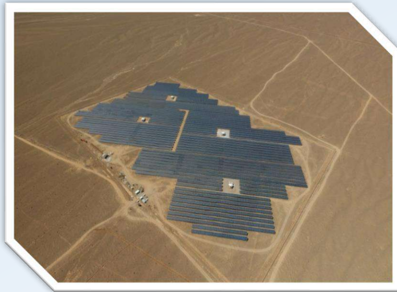
10 MW capacity grid-connected PV power plant (Fars, Iran)
