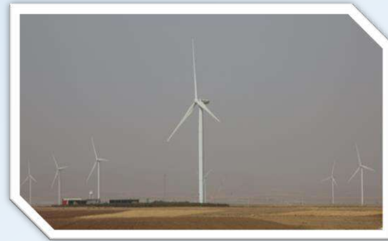
55 MW Wind farm (Takestan, Qazvin Province, Iran)
