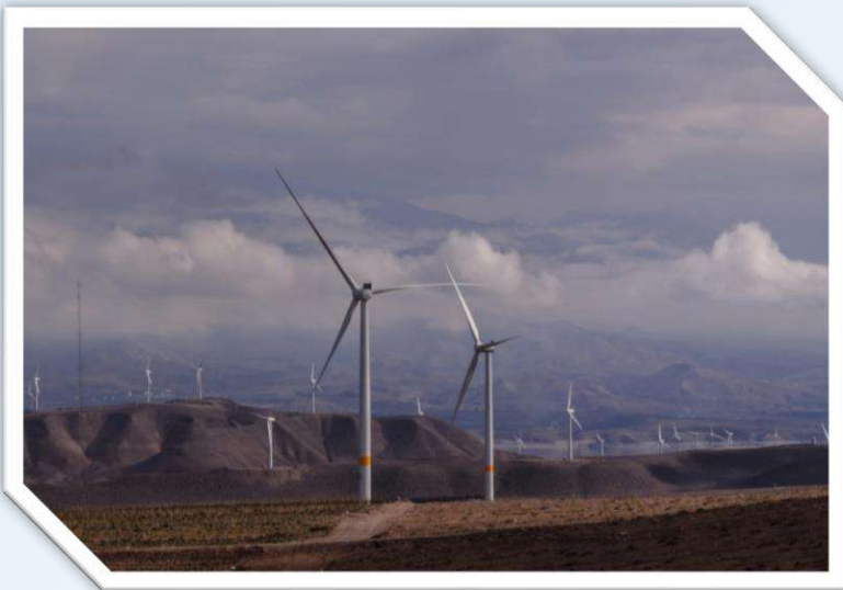
61.2 MW Wind farm (Qazvin Province, Iran)
